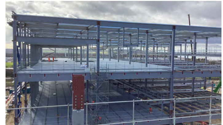
Envision AESC manufacturing facility – under construction
