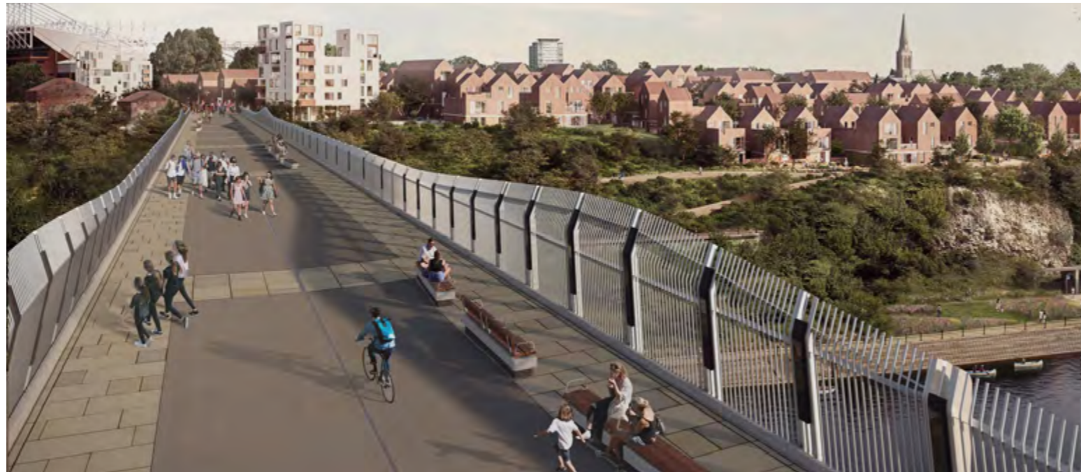
New Wear Footbridge, connecting Riverside Sunderland
