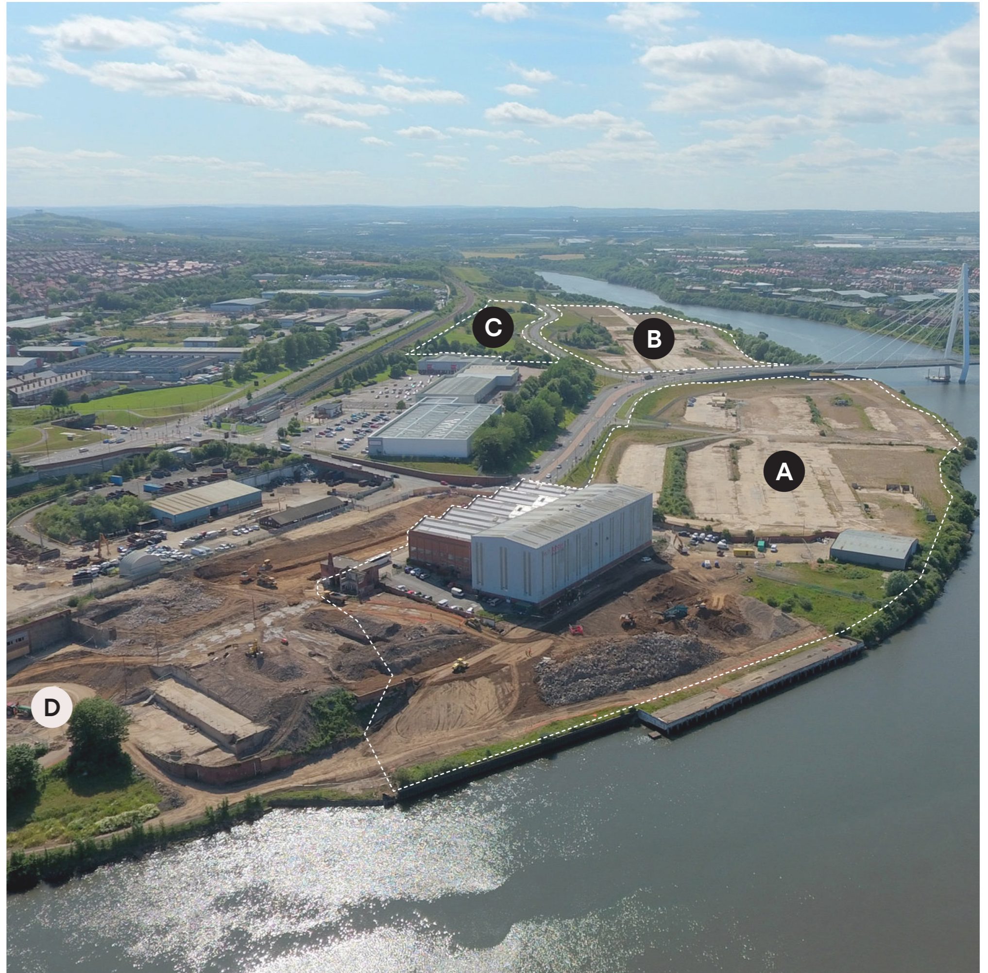
Crown Works Aerial - [Credit: SSTC3 asbestosaudit.com]
